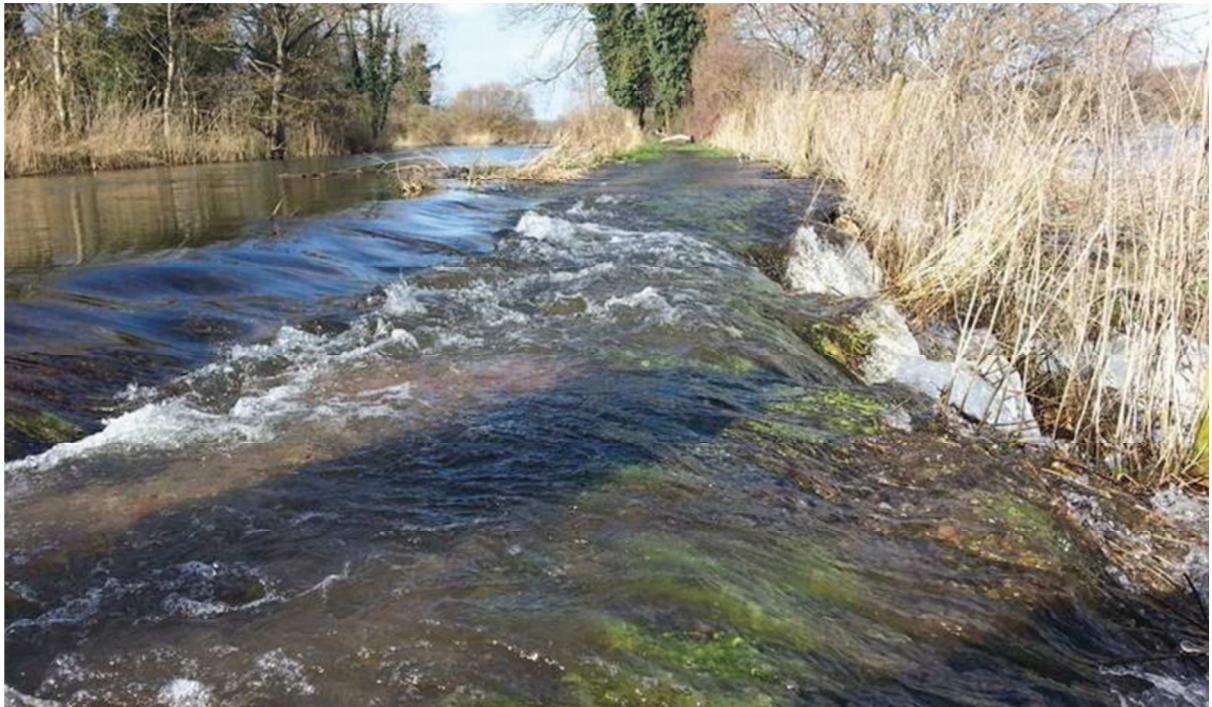
Figure 3: Flood Damage and Overtopping, Burghfield
